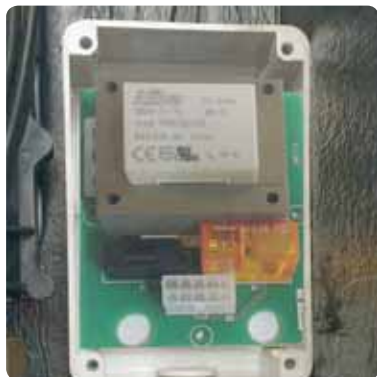
Figure 60 Thermostat-Relay box terminals Combi boiler
