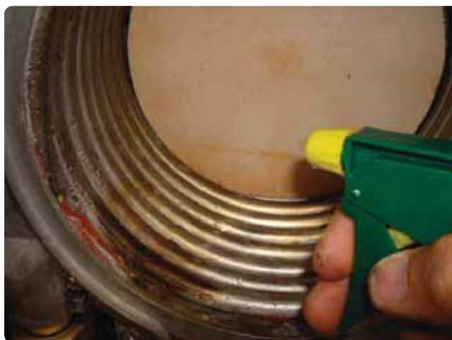
Figure 115 Cleaning the heat exchanger
