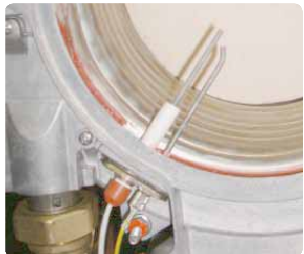
Figure 106 Inspecting ignition electrode
