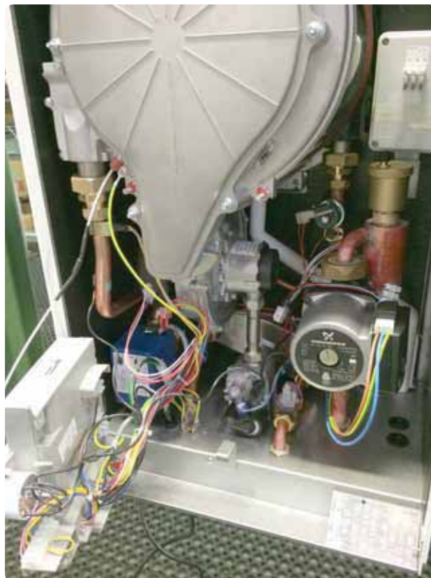
Figure 109 Boiler front panel removed
