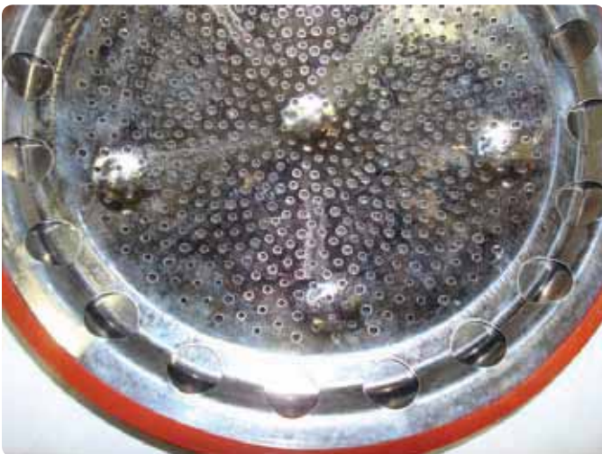
Figure 112 Inspecting interior and cleaning the burner
