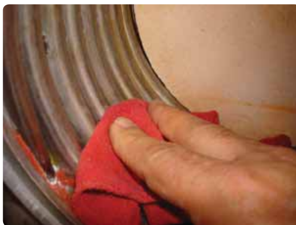
Figure 117 Cleaning the heat exchanger
