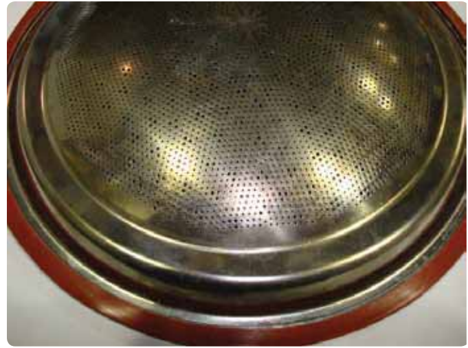
Figure 113 Inspecting exterior and cleaning the burner
